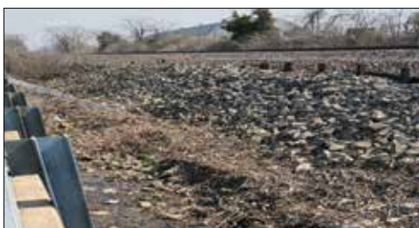
Stober Road ditch project completed.
