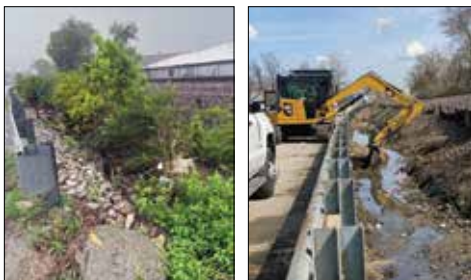
Stober Road ditch before clearing. Stober Road ditch clearing in progress.
